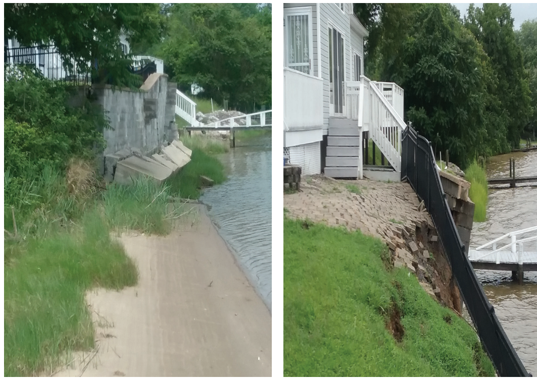
Unstable Retaining Wall and Eventual Collapse Due to Erosion
